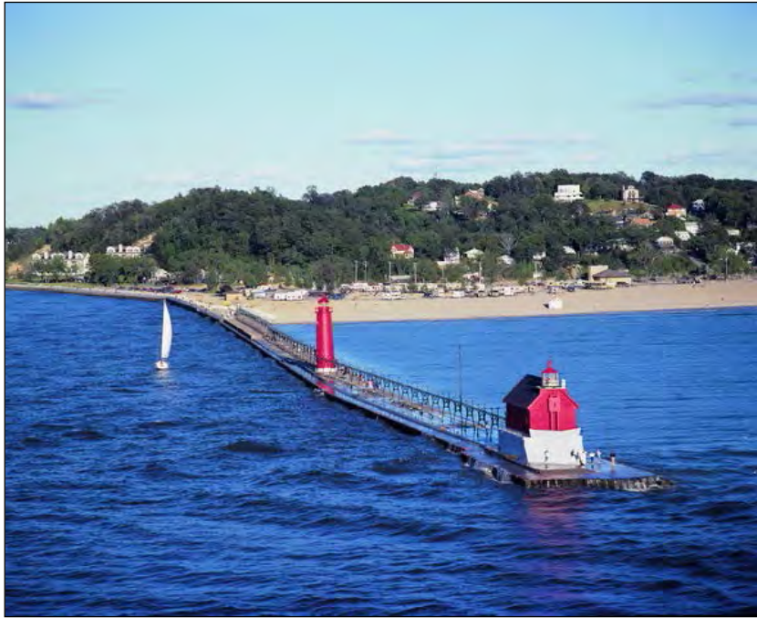
View of South Pier, Entrance light, Inner Light and Catwalk, Grand Haven, Michigan, July 2011. Photo credit: Aerial Photography, John L. Wagner, East Lansing, Michigan.
