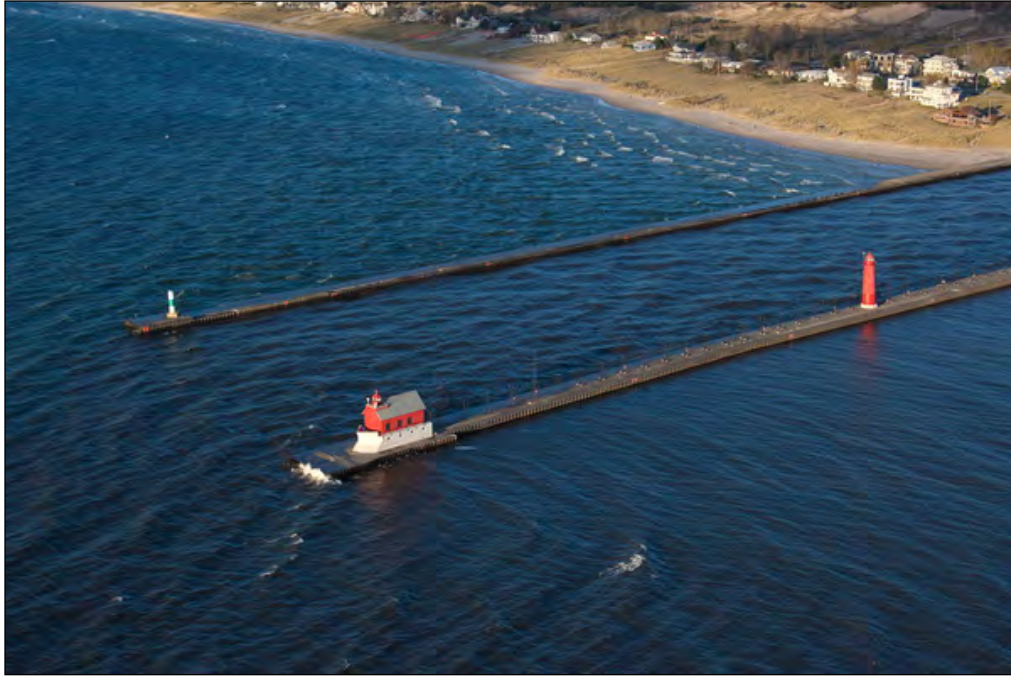
View of North and South Piers, Grand Haven, Michigan, October 2008. Photo credit: Aerial Photography, John L. Wagner, East Lansing, Michigan.
