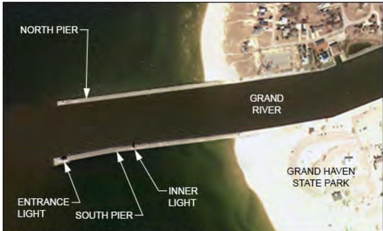
VIEW #1 - NORTH AND SOUTH PIERS
