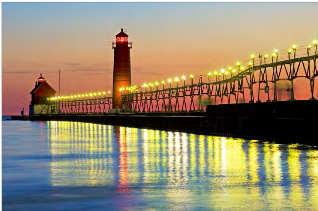
View of South Pier, Inner Light, Entrance Light and Catwalk illuminated at dusk, Grand Haven, Michigan, July 2007. Photo credit: Lake Superior Photo, Marquette, Michigan.
