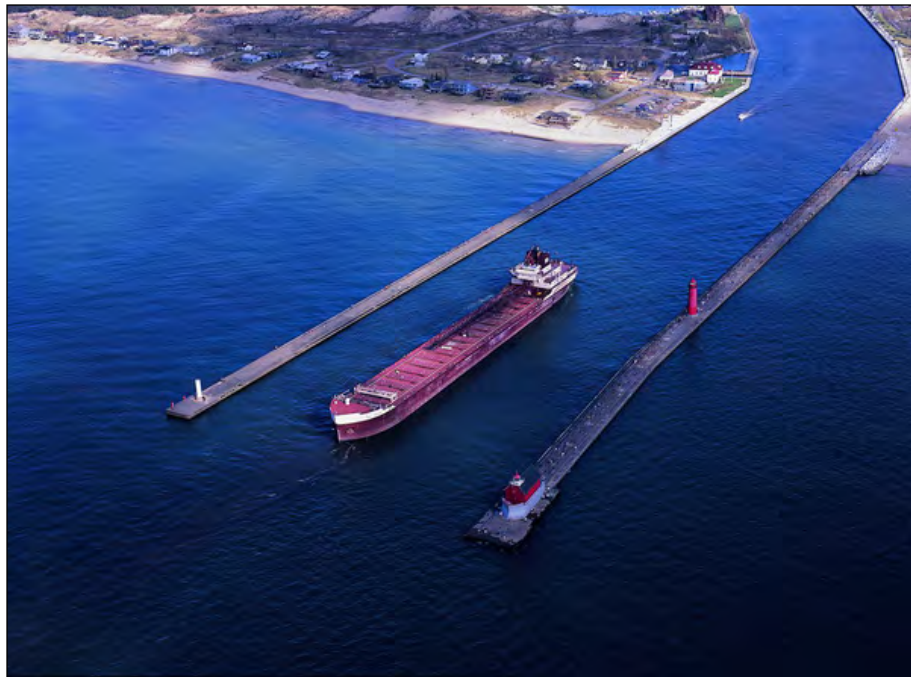
View of North and South Piers, Grand Haven, Michigan, July 2011. Photo credit: Aerial Photography, John L. Wagner, East Lansing, Michigan.
