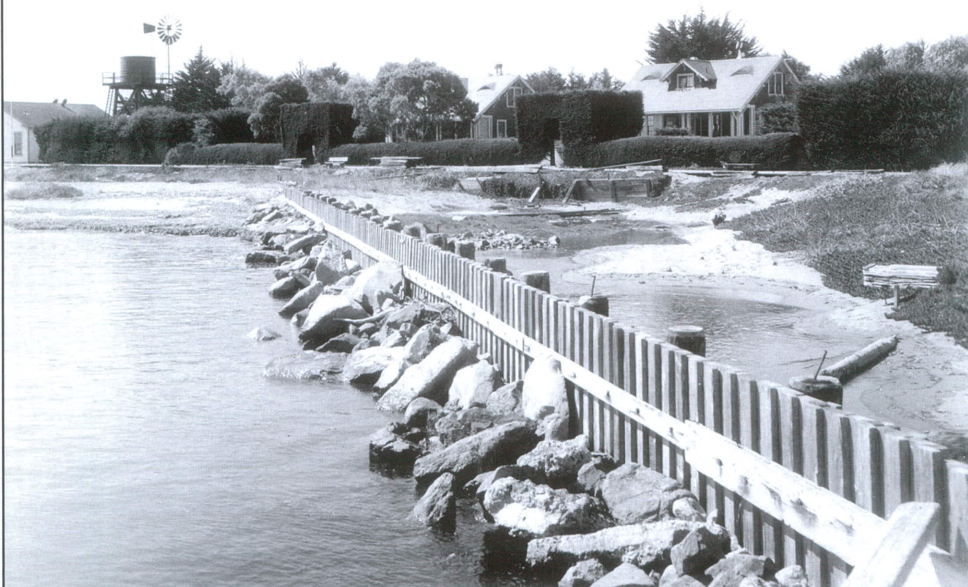
Humboldt Bay Fog Signal Station. The fog signal building is on the left and the keeper's dwellings are on the right. This station was constantly threatened by the waters of Humboldt Bay and eventually discontinued. Circa 1930 photograph from U. S. Lighthouse Society archives.
