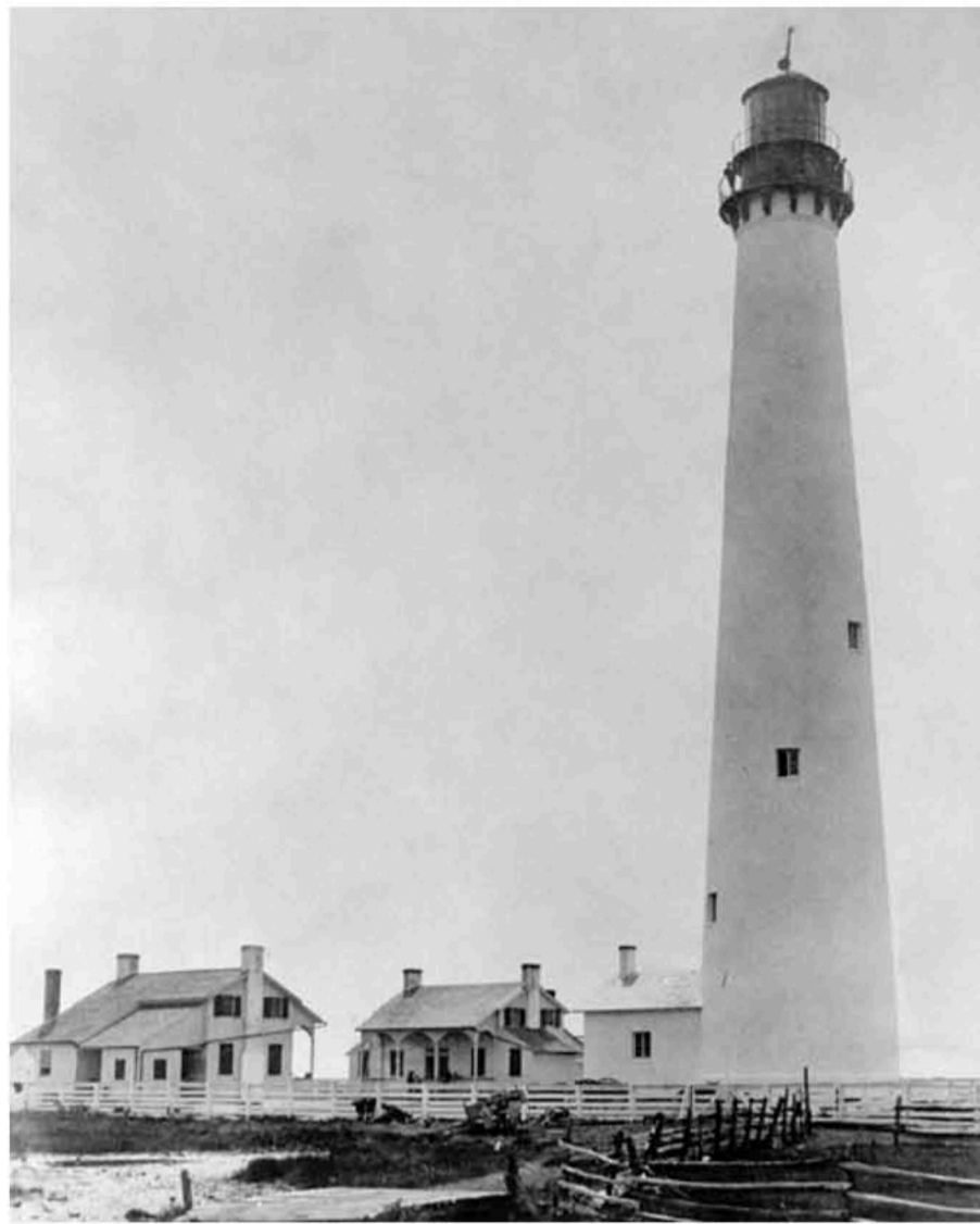
The second Cape Charles Lighthouse, completed in 1864 (US Coast Guard Historian's Office via LighthouseFriends.com)
